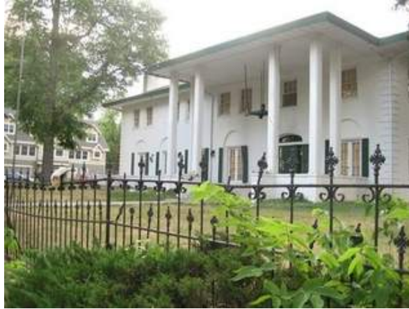
A developer is proposing to raze the boarded-up former Sigma Alpha Epsilon house at the corner of Howes and Laurel streets, across from the CSU Oval. (Trevor Hughes/The Coloradoan)
